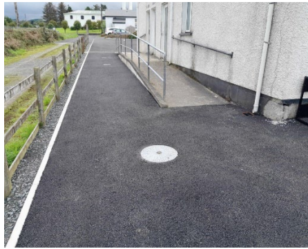
Fig. 9 Newly surface grounds and kerbs to front of the Clubhouse building
