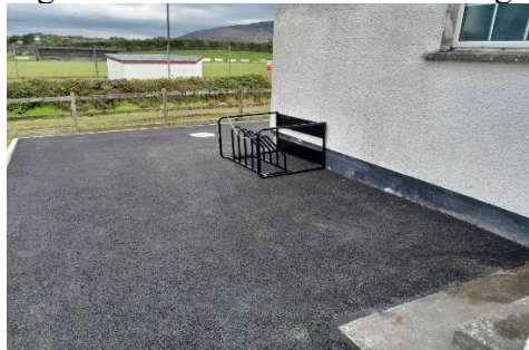
Fig.11 Newly installed bicycle rack to side of Clubhouse
