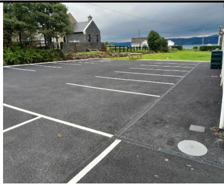
Fig. 8 Newly surfaced carpark, line marking and Aco-Channels.
